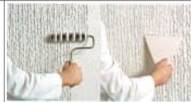
Capa-Rollputz is evenly applied with a smoothing trowel, then vertically rolled with a texturing roller and textured with the smooth side of the spatula (pressing offset and drawing slightly). Consumption: approx. 3400–3700 g/m 2 .
