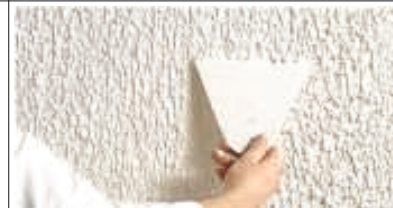
Capa-Rollputz is applied with a perforated styrofoam roller and then smoothened using trowel or spatula. Consumption: approx. 3200–3500 g/m 2 .
