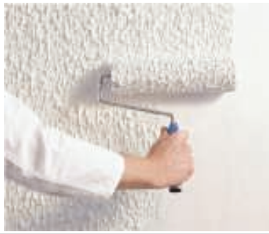
Application of Capa-Rollputz with a perforated styrofoam paint roller.
