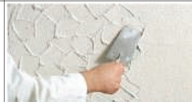
Even application with a smoothing trowel. Texturing is effected by pressing offset/staggered with the trowel and drawing slightly. Consumption: approx. 3400–3700 g/m 2 .
